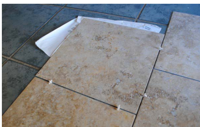
Fig. 1 - Use spacers to maintain the joint width
