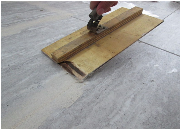
Fig. 2 - Pack the grout into the joints
